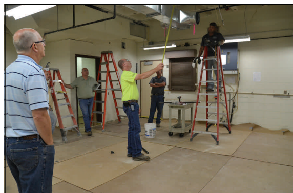
Dr. Nowack looks on as the crew installs our high-volume air handling system in the 3rd floor stockroom.
