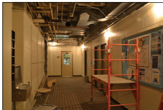
Ceilings were removed to allow all ductwork to be upgraded. New wiring for an alarm system was also installed.
