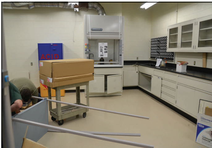
Showing new flooring, new counter top, and new fume hood. In the foreground, the new shelving units are being assembled.
