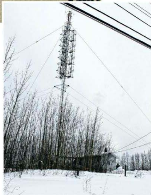
VOAR tower in Prince George, B.C.
