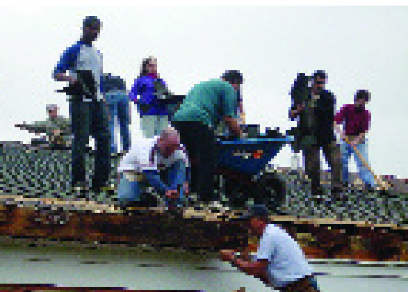
Volunteers from the Williamsport (Md.) church repair and re-shingle the roof of HVA's administration building.
