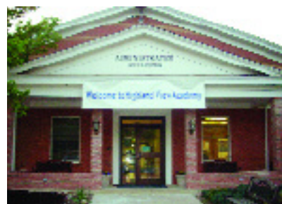
The new administration building entryway is partially completed.
