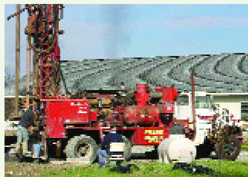
The Frame Drilling Company works on hole number 5 for Highland Adventist School's new geothermal heating and cooling system.
