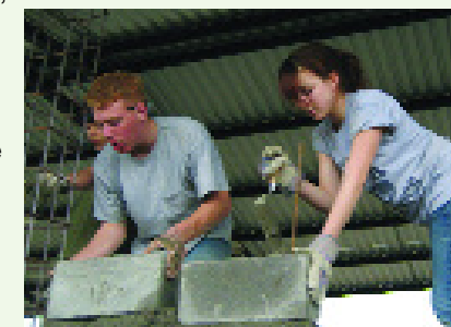
Sophomore Nathaniel Bankes and junior Mary Hostettler help lay bricks for the new auditorium/multipurpose room of Instituto REACH Internacional.
