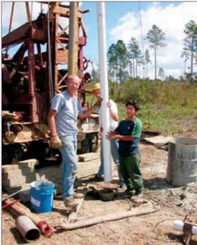
Gary and Rod Bartholomew and Donaldo Lopez work on the well.
