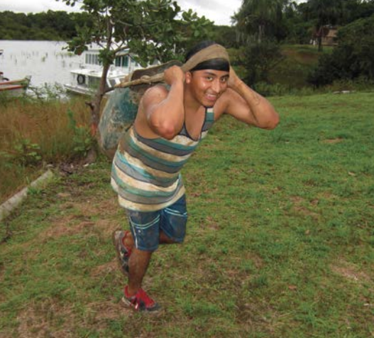
Junior Moises Ramirez uses local methods to move dirt for the clinic's foundation.
