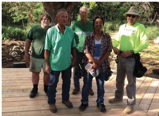
(L. to r.) Guy Smith, Norman McGuire, Patrick McGuire, Robert Lacquia, and Rod Seibel work together to build the new Tree Chapel stage.
