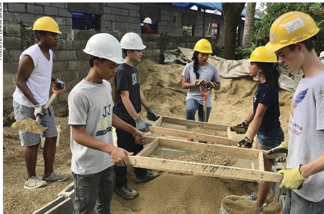
Carmichael youth and a local Dominican teenager prepare concrete by sifting and mixing cement and sand at the Villa Mella church construction site.
