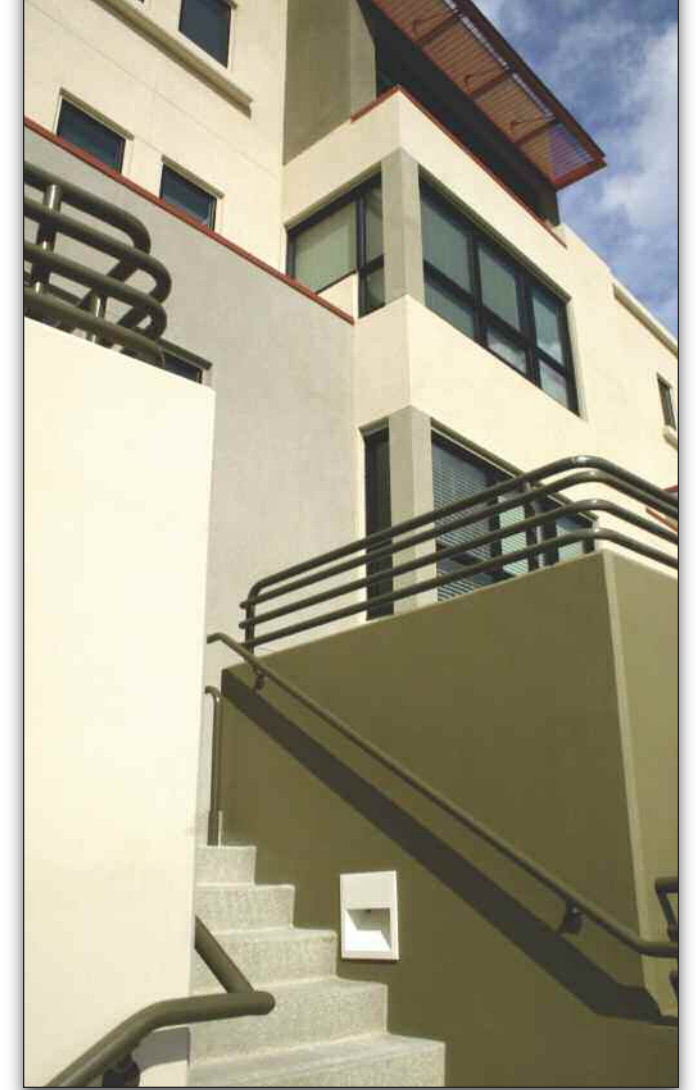
Campus housing has been a challenge for Loma Linda University students. This addition provides some much-needed housing facilities. ▲
