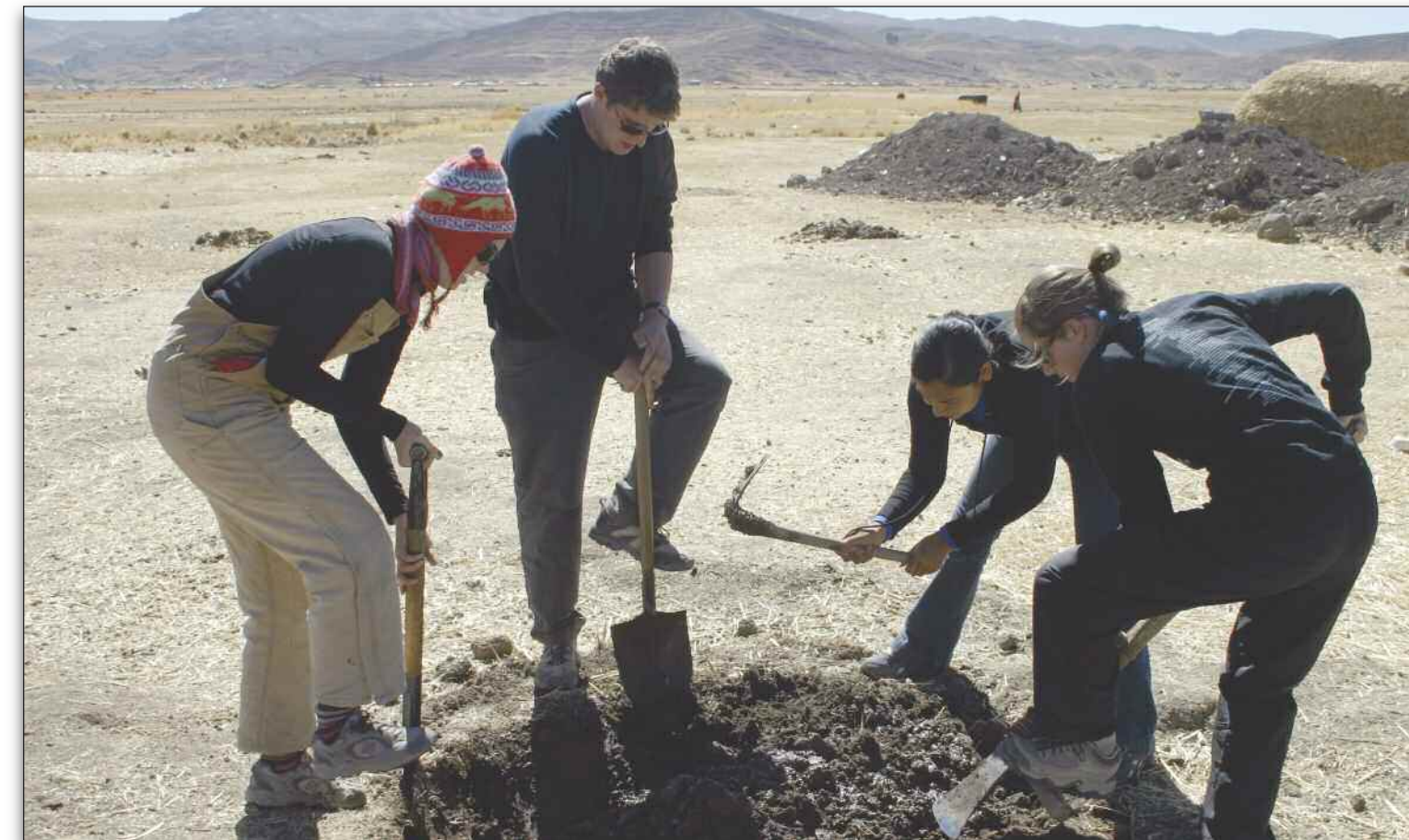
(From left) Nikki Grey, Dana Johnson, Rebecca Medina, and Jamie Goyette prepare earth for use in the construction of a cobertizo, or cattle shelter. ▼
