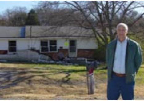
Roy Shouppe stands in front of the house where the water heater exploded.
