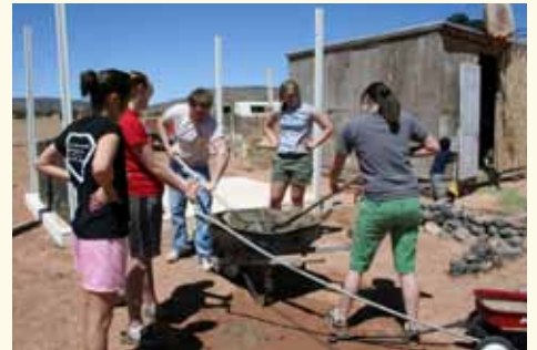
Seniors mix mortar needed to repair an outdoor oven for an elderly Navajo Indian.
