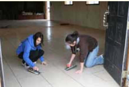
Rachel duBois (left) and Laura Cole grout the ceramic tile that the seniors laid for a local church in Holbrook, Ariz.
