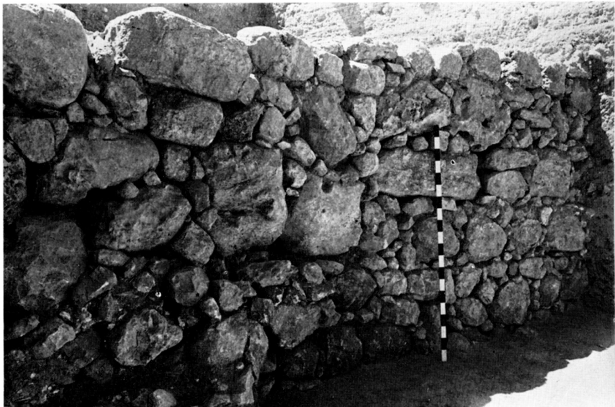
B. Area B: north face of Wall 17B of the Persian period. The foundation, lying deeper than what is visible in the picture, was not reached in the 1968 season
