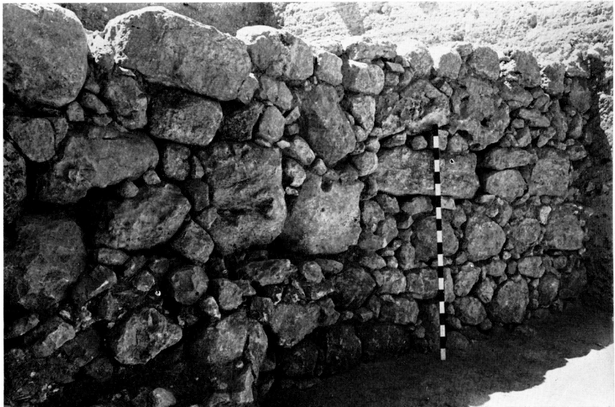
B. Area B: north face of Wall 17B of the Persian period. The foundation, lying deeper than what is visible in the picture, was not reached in the 1968 season
