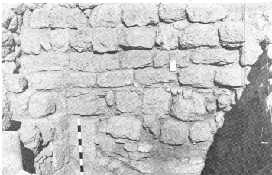
B. East face of Wall D.6:3. Phase 3a comprises the top five courses and the fill in the blocked doorway beneath the white tag. Phase 3b is represented by the doorway itself, while Phase 3c is the step at the bottom
