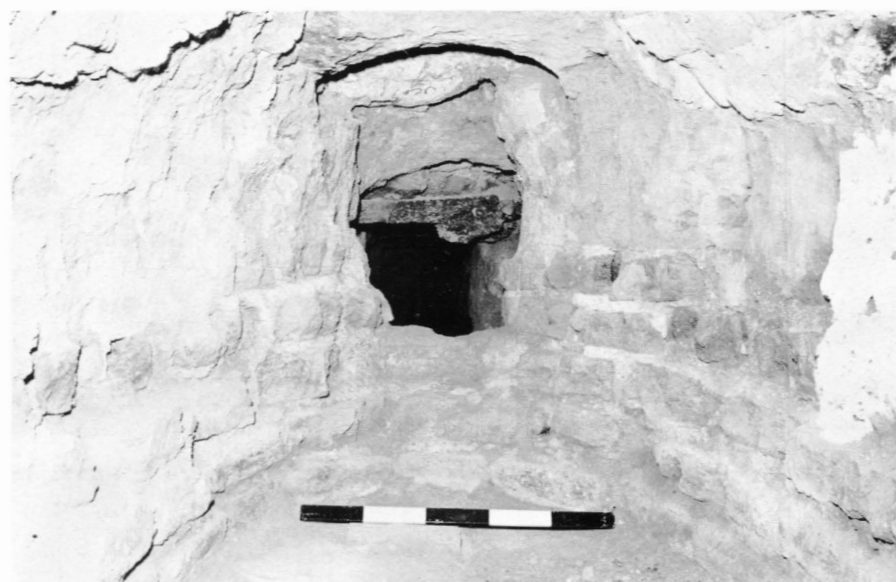
B. The inside of the furnace looking toward the horizontal flue which begins at the hole in the background. It heats the bathing room above. The edge of a black basalt slab is visible on which the floor tiles rest. Photo: Avery V. Dick.
