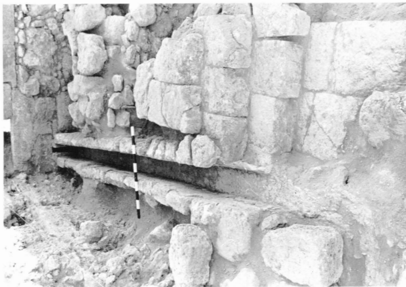
A. Water Channel D.1:58 = D.2:30 running from beneath gateway through Wall D.1:4c in the background to Stairway D.2:32 (on right), Stairs D.2:7b (on left), and Stairs D.2:34 (bottom left). Photo: Avery V. Dick.
