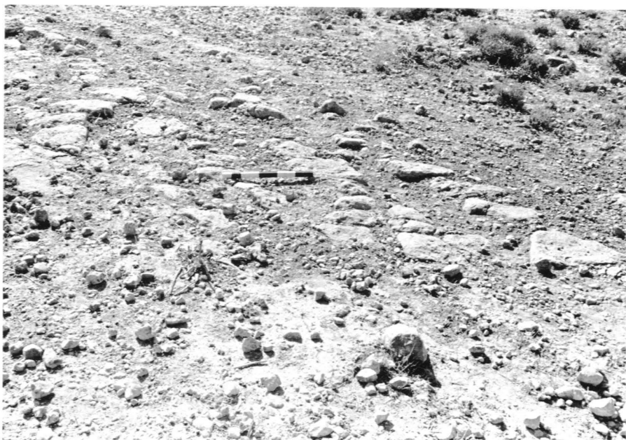
A. Cobble stones of the Roman road east of Site No. 35 (Grid Reference 2196.1341). Photo: Avery V. Dick.
