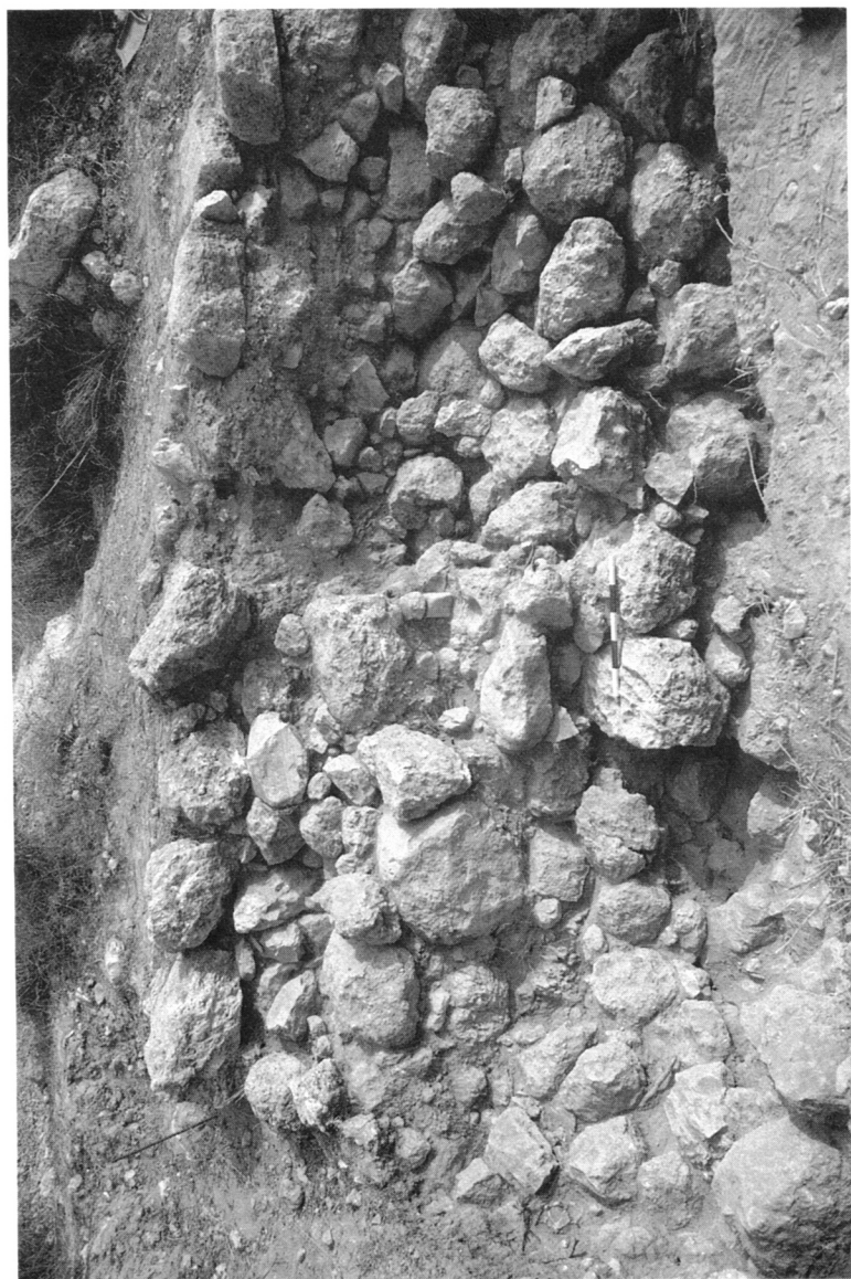
Plate 11. Two phases of Outer Wall; meter stick rests on earlier phase.
