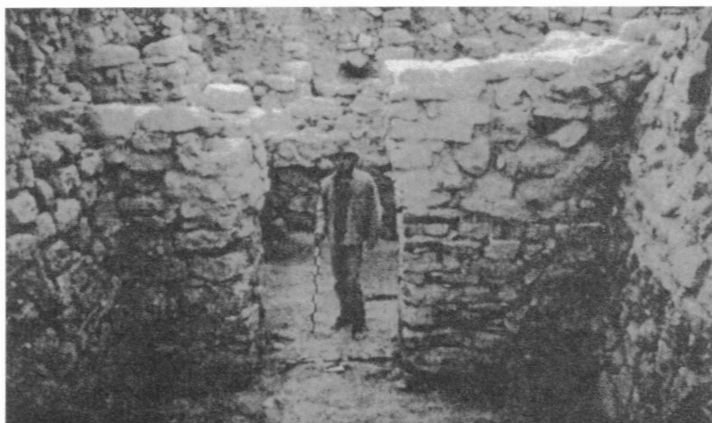
Figure 7. Tall al-'Umayri: Looking from the western room of the LB building in Field B through the door, illustrating the excellent masonry and preservation of the walls. The upper courses were consolidated with cement in 1998 to protect the walls from destruction.
