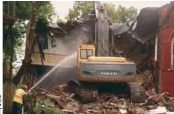
City equipment demolishes a portion of Utica, New York's Karen Adventist Church building to access collapsed sewer pipes for repair.
