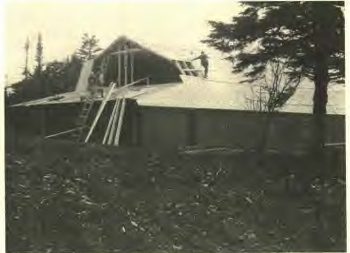
Platform end of building.
