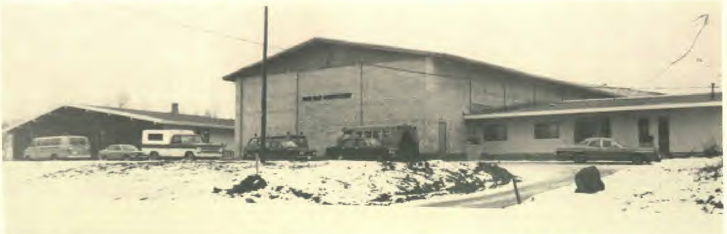
Fraser Valley Adventist Academy showing elementary section, gymnasium, and secondary school section.
