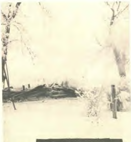
The scene of the fire in Acme, Alberta on January 4, 1977.
