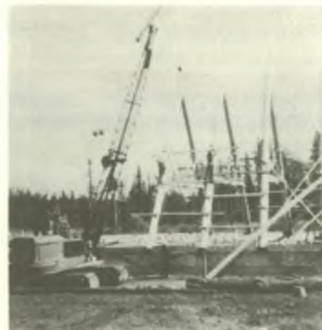
Log "A" frame beams going into place.
