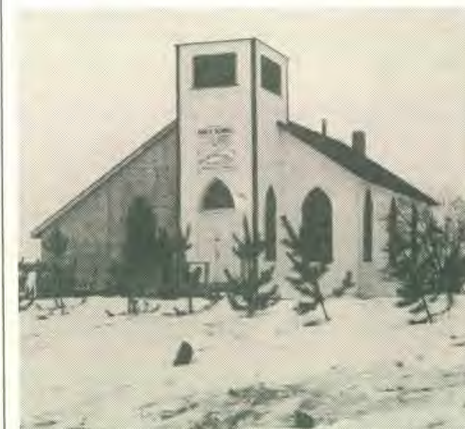
The church at Hobbema with the new addition for mother's room and washroom facilities.
