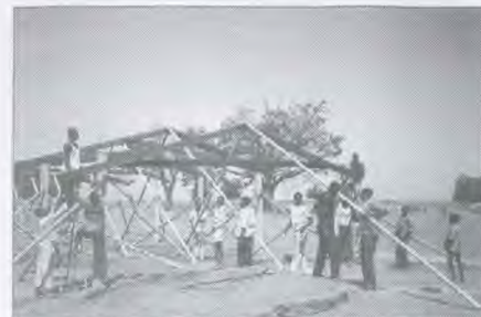
Construction of a school/church building
