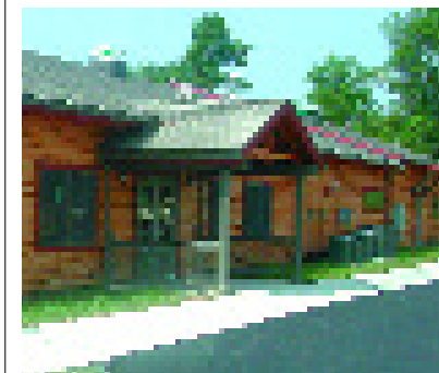
The new Pine Forge Elementary building was funded with a CURF loan.
