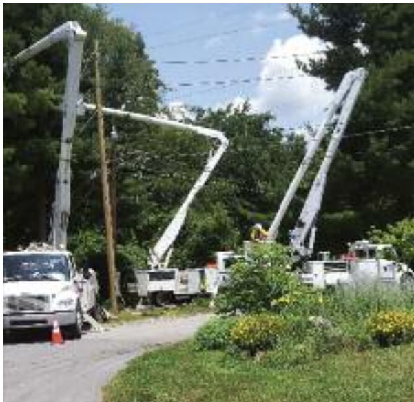
Out-of-state electrical technicians work to restore power.
