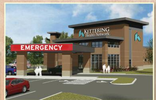
Groundbreakings held for freestanding Emergency Centers in Springboro/Franklin and Preble County.
