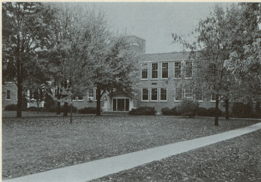
Nethery Hall is one of the name places on AU campus. It honors J. J. Nethery, former board member of Andrews University (then EMC).
