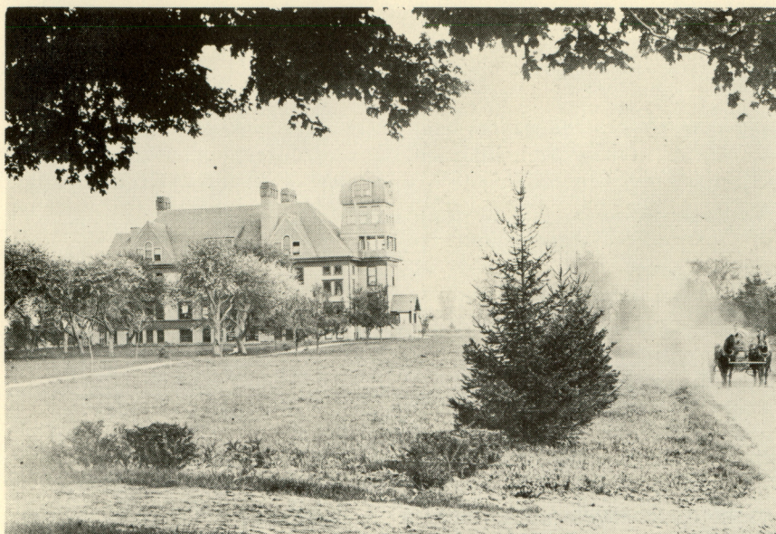
The first administration building at EMC was built in 1903 at a cost of $8,000 for lumber. It was converted to a dormitory in 1943-44, after a new administration building had been completed, and continued in use until it was torn down in 1953.
