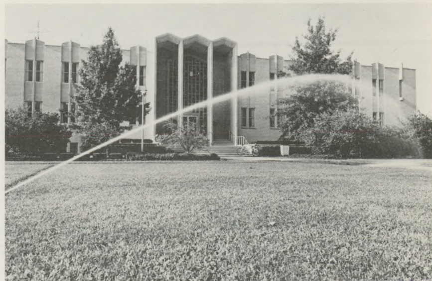
New sprinkler head, part of the $15,000 system at Andrews University, shoots water on grass near Seminary Hall. The system is to be extended to cover the entire campus within five years.
