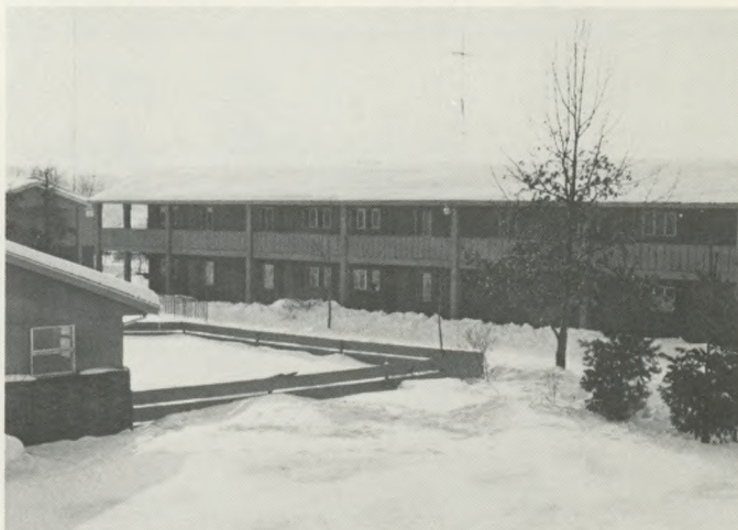
A portion of the Rose Hill Manor apartment complex leased by Andrews University.
