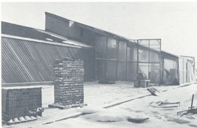
February progress on the exterior of the new Heritage Bank.
