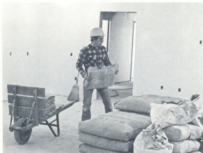
February progress on the interior of the new medical center.
