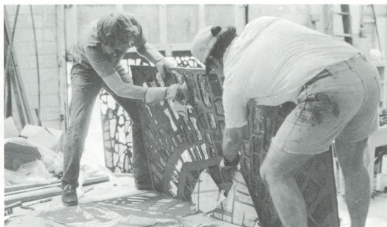
Ty Leinnewebe, a junior architecture student, and Bill Belles removed the paper pattern after allowing the panels to dry for six hours. Total drying time was two weeks. Each panel weighs about 150 pounds.
