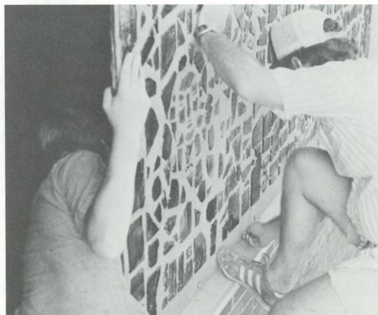
In spite of their size and weight, each of the 46 panels is secured only by steel screws at the top and bottom.
