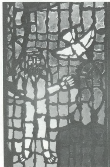
In spite of their size and weight, each of the 46 panels is secured only by steel screws at the top and bottom.
