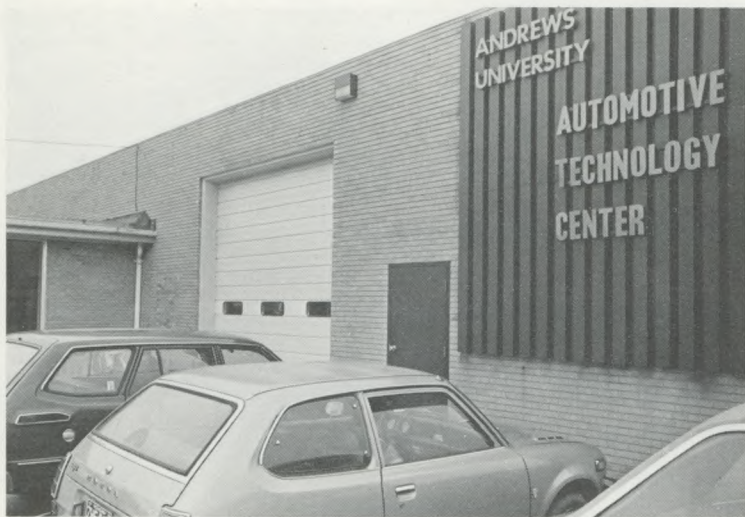
The renovation of an 8,900-square-foot facility on Highway 31-33 in Berrien Springs houses the expanding automotive technology programs in auto body and auto mechanics. This provides an adequate facility at a more visible location to the general public.
