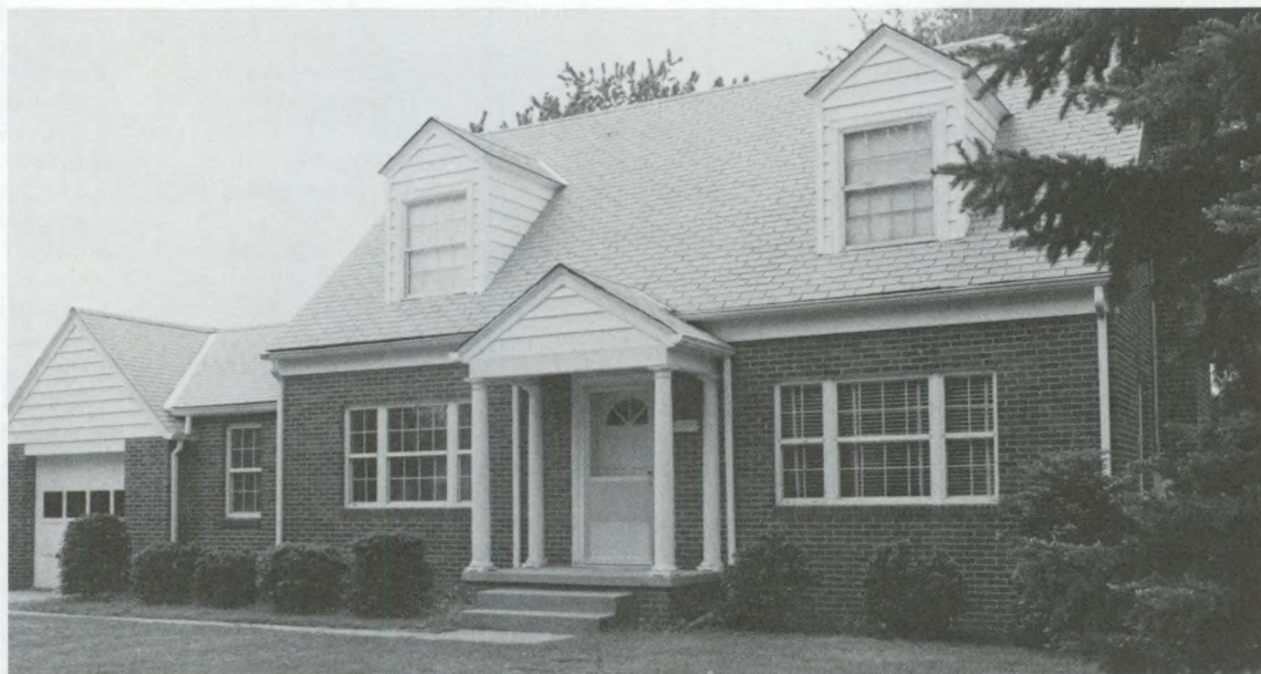
The new offices for the Alumni Association, located at Seminary Drive and Grove Street, will house administrative offices, computerized alumni records and an alumni lounge.
