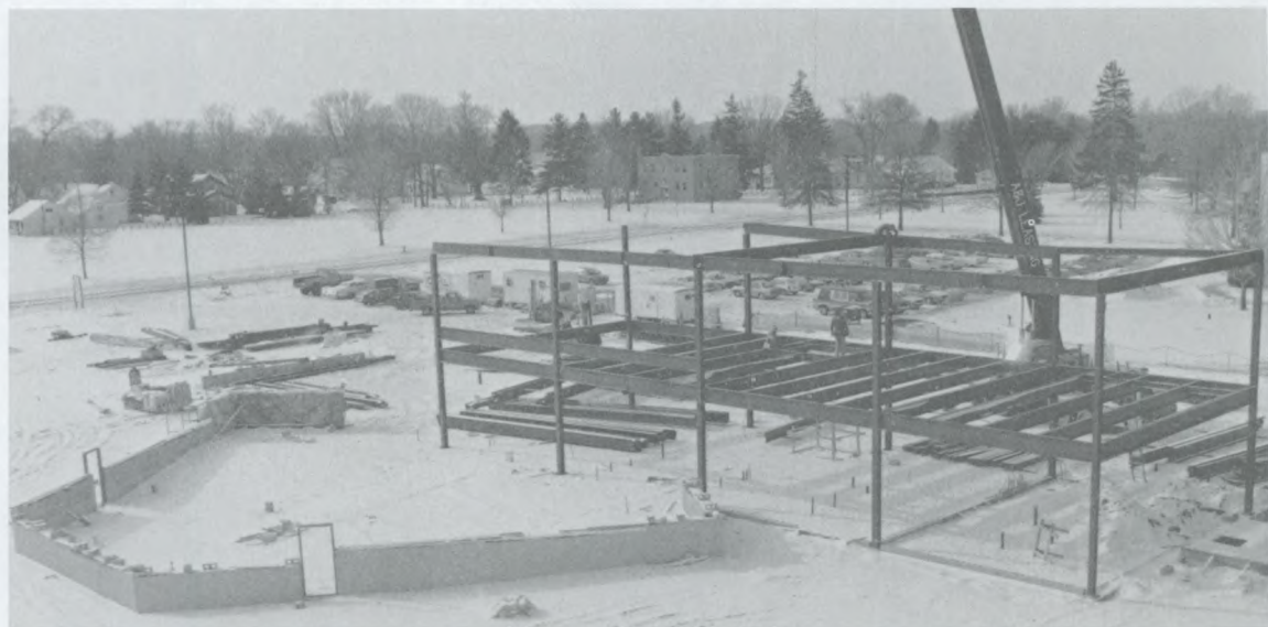
Amid snow and rain, the new School of Business building took shape during fall quarter. The building, to be named Chan Shun Hall after a Hong Kong businessman who was a major investor, is scheduled for completion by the fall of 1989.
