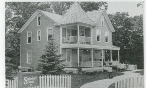
Photos from 1985, 1986 and 1987, show the restoration of the Sutherland House.
