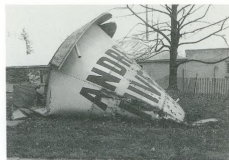
1987 The first of two water towers comes down.
