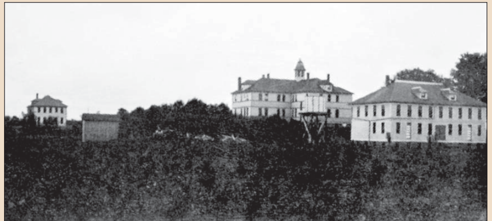
The rear view of the new campus buildings (1903). Advocate publishing office, Domestic Art Building, and Manual Arts Building (l to r)
