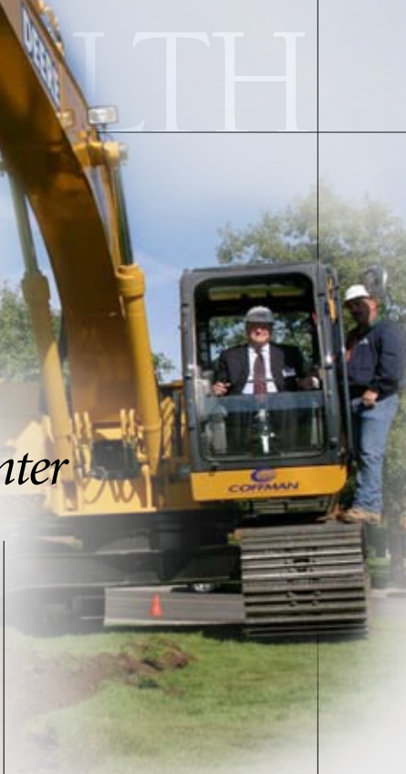
Deryl Jones takes a spin in the earth mover at the Pavilion groundbreaking event.
