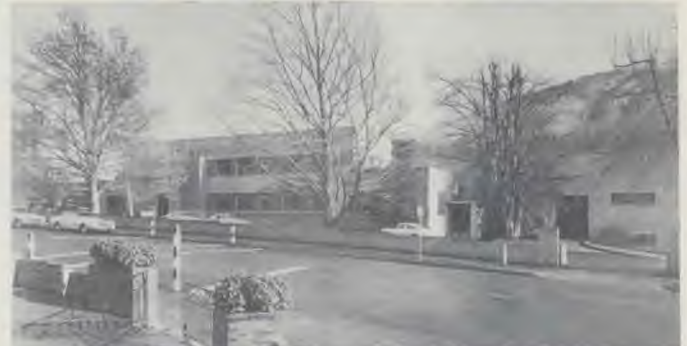
The present plant at Warburton, set in the beautiful Yarra Valley.
