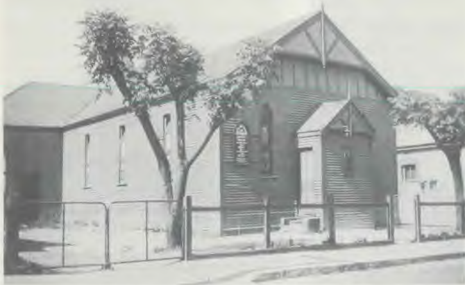
The original wood-and-iron structure built in Ballville Street by Prospect members in 1905. Photos: The late Lionel Brown
