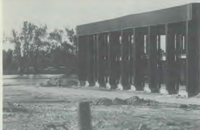
The office section, overlooking the nearby lake. Paving is now down.
