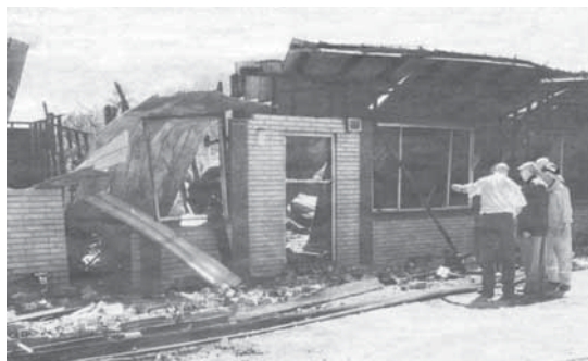
Detectives, Country Fire Authority members and church members inspect the remains of the church hall.
