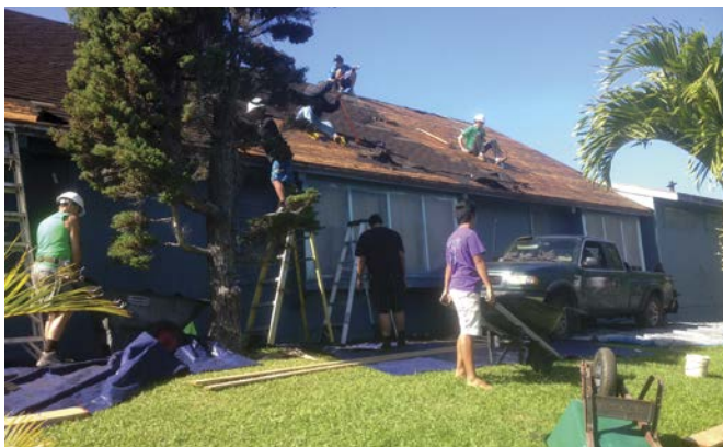
Volunteers remove the old roof in preparation for the new.
