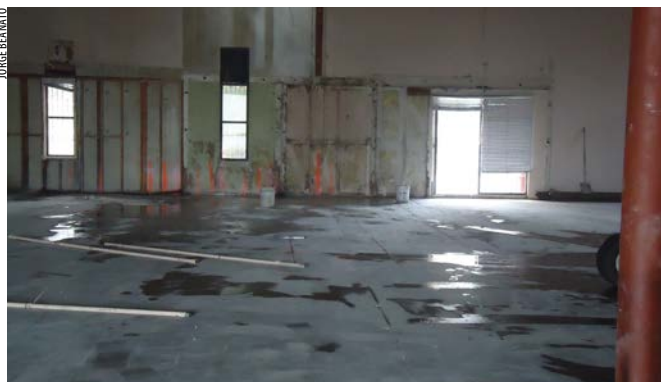
A former warehouse in a residential neighborhood required extensive renovation to become a house of worship.
