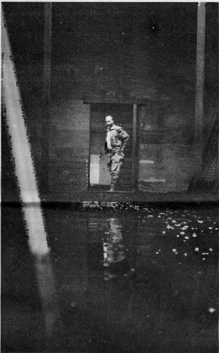
VERNON E. EVANS , Maintenance Service engineer, checks the cavernous interior of the air conditioning heat-exchange units, constructed of asbestos fibre materials and rot-resistant redwood.
