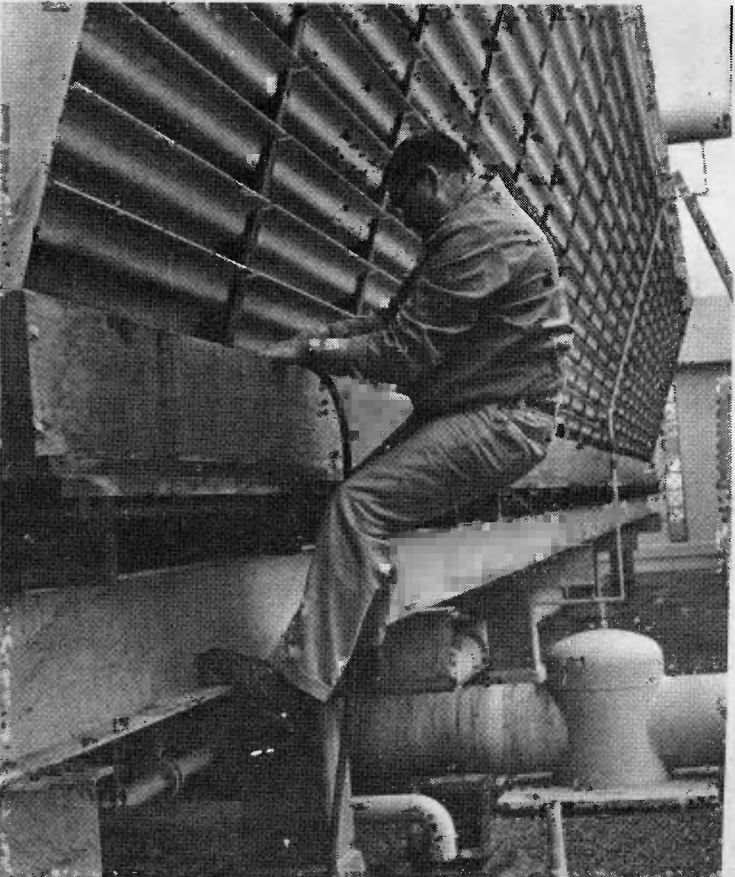
ASSISTING in the preparatory cleaning of the plant's air conditioning system "chillers," Roscoe A. Trunkey, Maintenance Service engineer, uses a hose to wash out sediment.
