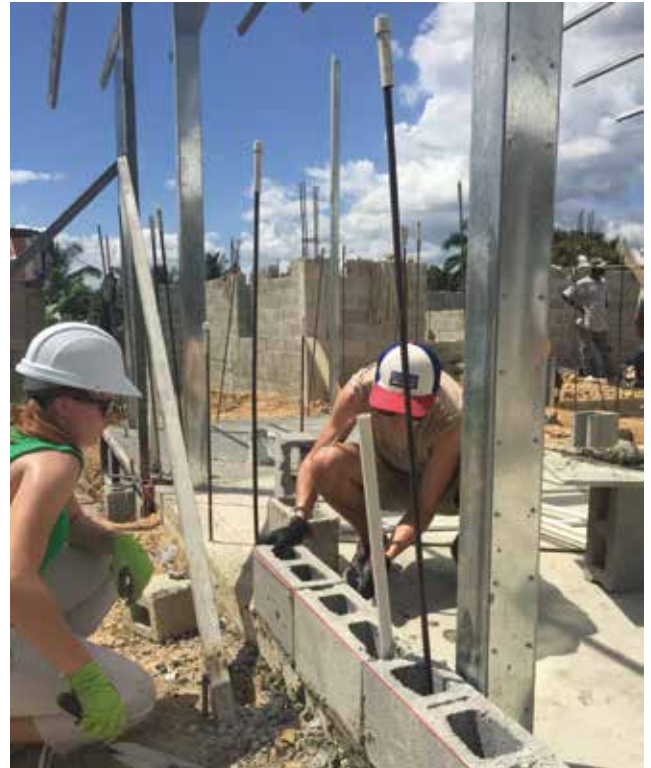
Avery Kroll, senior, and Jackson Webb, junior, lay blocks for the Sabbath School building.
