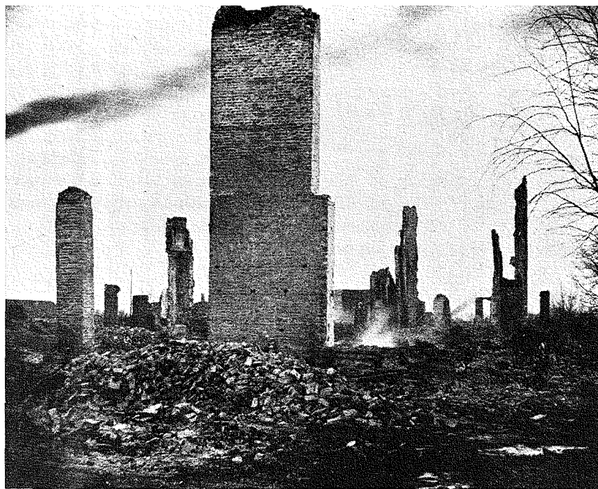
All that remained of the 1878 Battle Creek Sanitarium after the fire of 1902.
