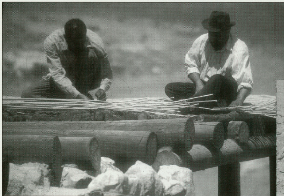
Clockwise from left: Application of reeds into roof structure, laid across wooden branches. Below: Mohammad moving stone for household reconstruction. The manufacture of replica mud bricks for household construction.
